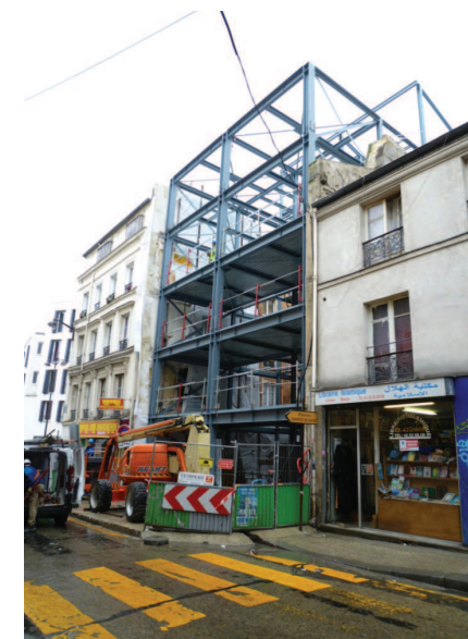
Façade sur rue (Nord Est) - Structure métallique achevée © North by Northwest
